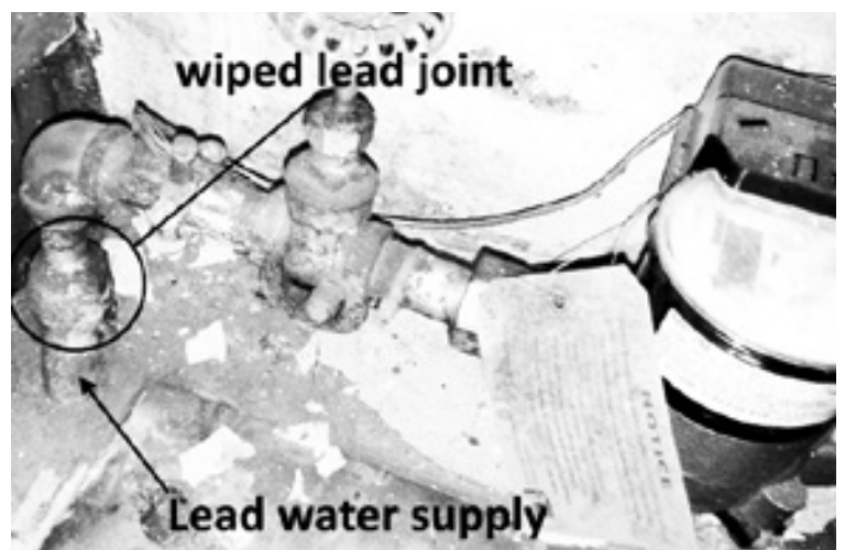
To accomplish the mandate to identify all homes with lead water pipe connections, all homes in Woodsboro built before 1973 will have to be entered to inspect connections to the Town's water system.
