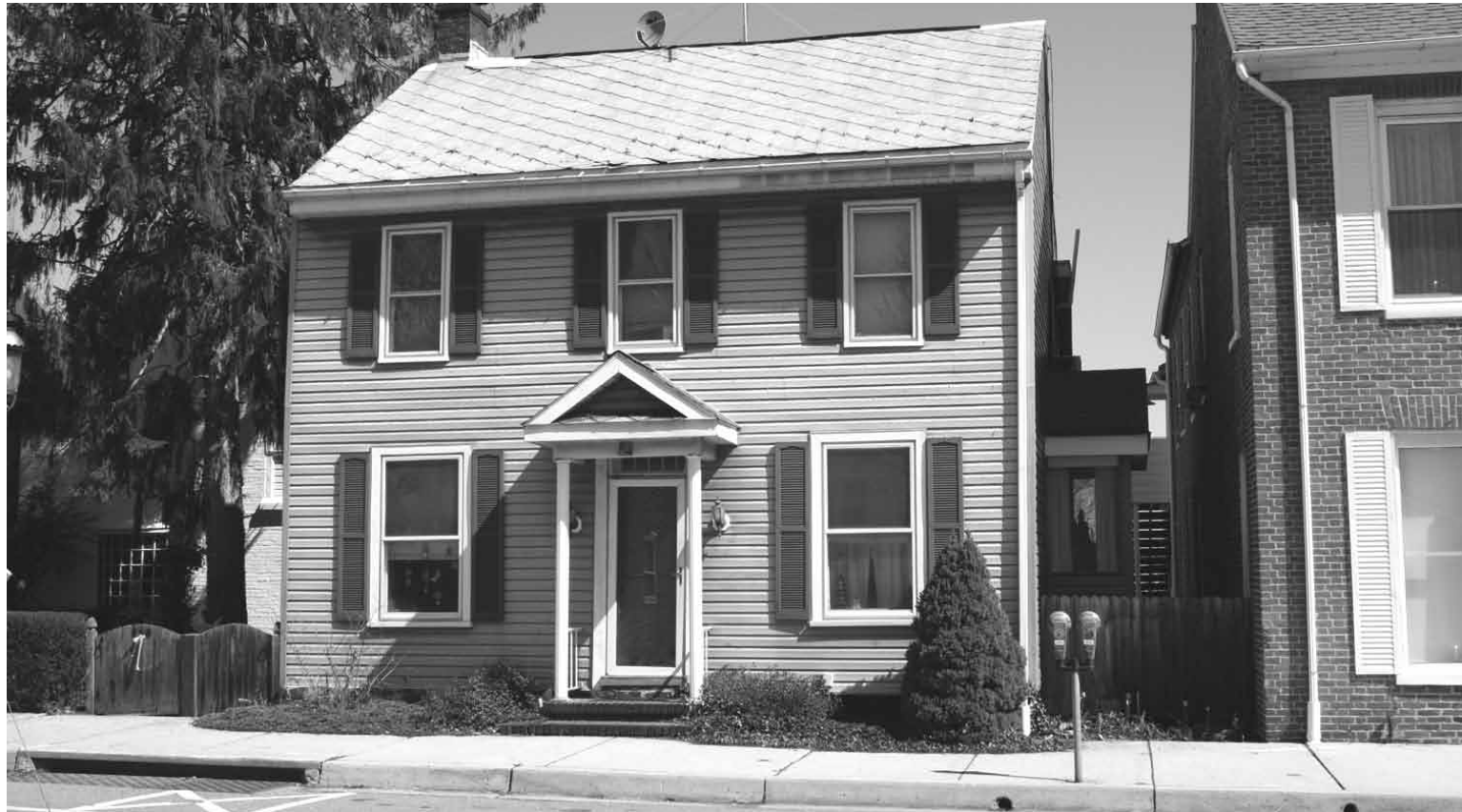
Location of the old phone office. Operator switchboard was in the downstairs room to the right.
